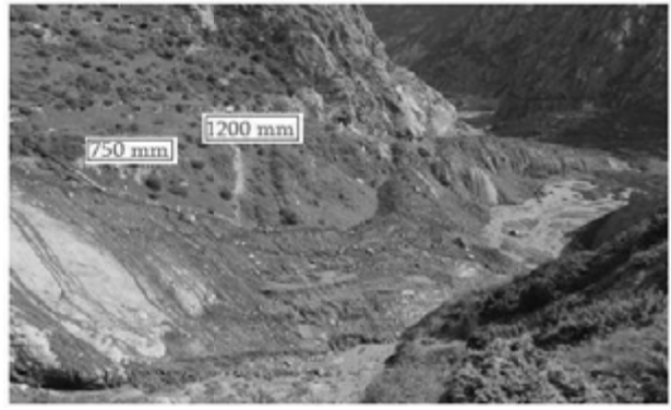
Fig. 2. General view of the demolished 1200-mm diameter and 750-mm-diameter Russian-Armenian gas pipelines running across the bed of the river Kabakhi as a result of mudflow
