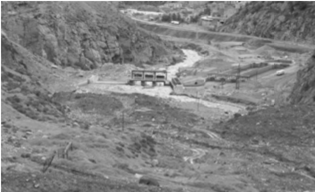
Fig. 3. General view of the hydraulic facilities of Daliari HPP under construction in the gorge of the river Tergi after the mudflow
